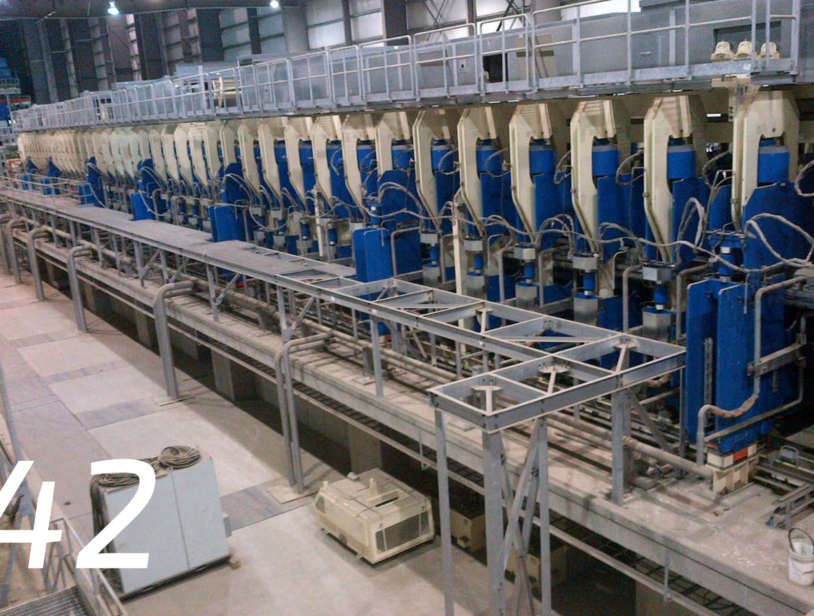
Pressendemontage in Grande Prairie, Kanada
